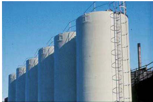
Figure 8.6 Storage tanks of malt vinegar after acetification
